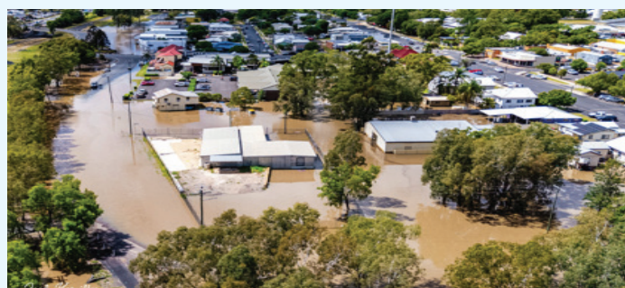
Impacts of floodwaters in Chinchilla
