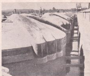
A close view of volute siphons for the automatic release of surplus flood supplies at the Havtkegar Dam.
