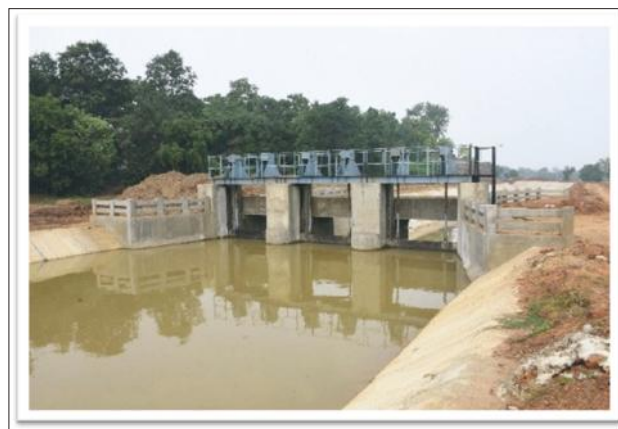
Pic-4. Cross Regulating Structure
