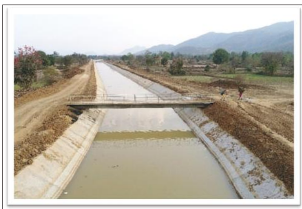
Pic-8. Walkway Bridge
