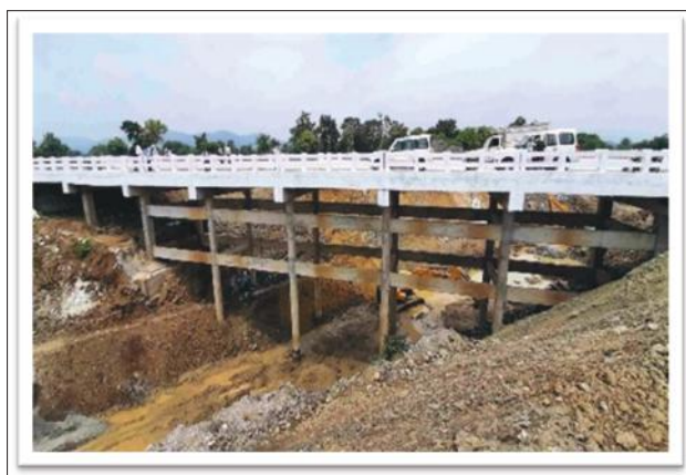
Pic-6. Village Road Bridge
