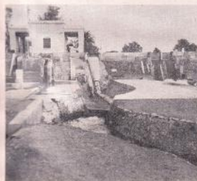
Model tests in connection with the Bhakra-Nangal Project at the Hydraulic Research Station, Malikpur. The facilities available at the station enable the construction of large scale river models.
