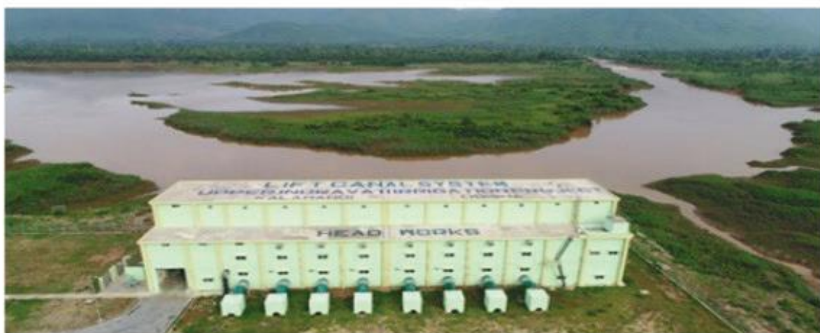
Pic-2. Pumping Station
