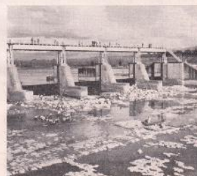
Handworks at Hardwar—Built in the middle of the nineteenth century and remodelled in 1917-20. The Ganga Canal taking off has a capacity of 8,400 cusec and irrigates 1.6 million acres annually.
