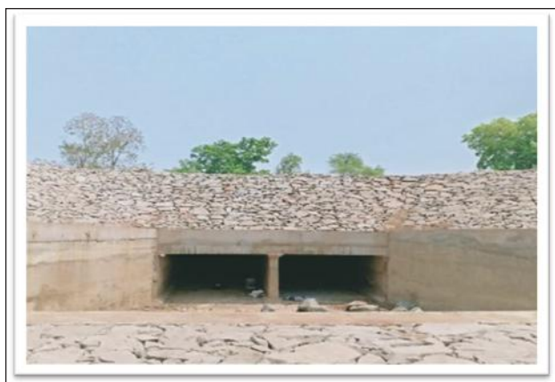
Pic-5. Cross Drainage Structure
