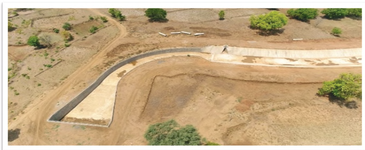
Pic-1. Delivery Chamber
