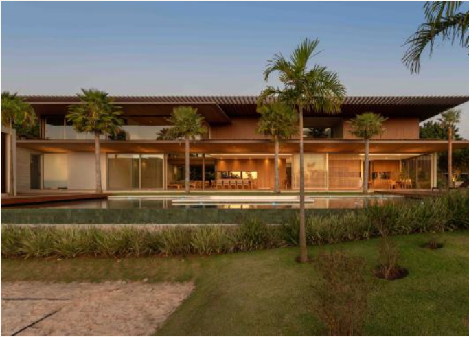
Rear façade and garden
