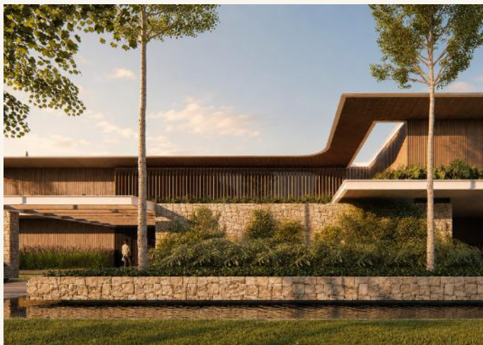
Main façade and landscape design
