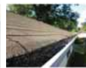
Roof & Gutter Maintenance
