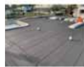
All Membrane Installation
