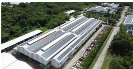
RAMCAR BATTERY PLANT
