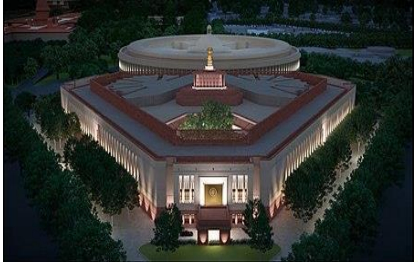
2022: New Parliament Building, New Delhi (under construction)
