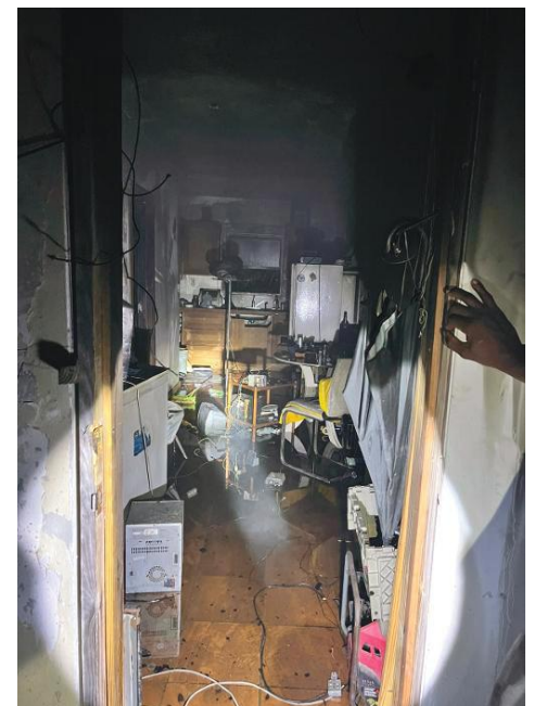
Photo shows a section of the house in Blue Hills that was affected by fire
