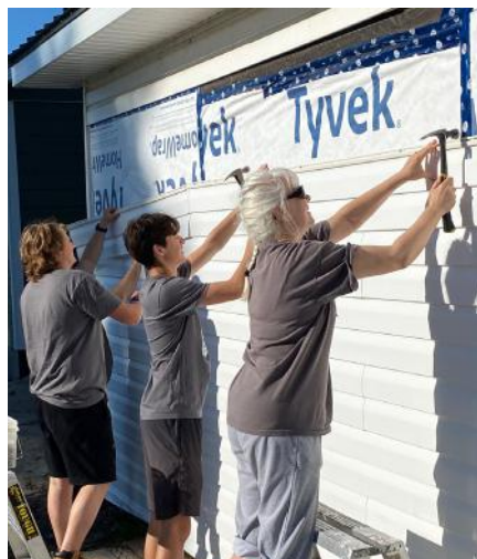
Installing vinyl siding was one of many tasks the group performed.
