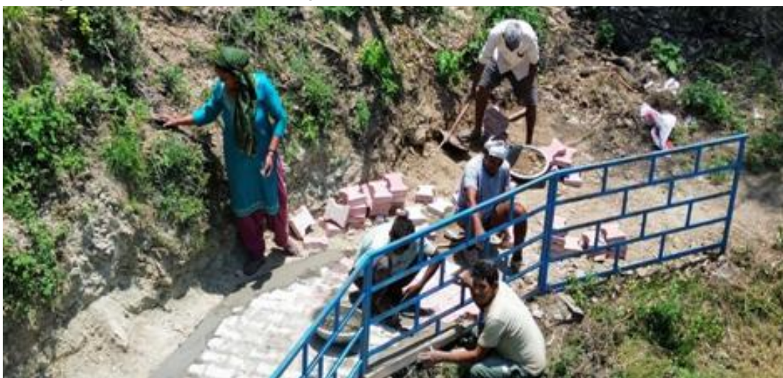
Shobha Devi personally supervising interlocking road construction work. (Source: Padma Award nomination document, personal collection)
