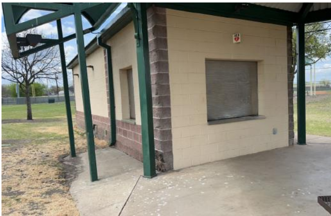
Independence Park West: Concession Building
