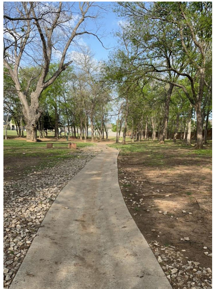
Freedom Dog Park: Drainage Concrete Channel
