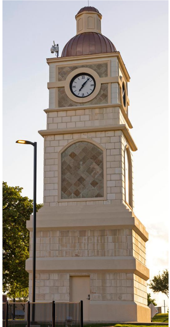
ToTC Clock Tower
