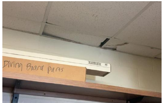
Independence Park East: Community Pool Storage Room
