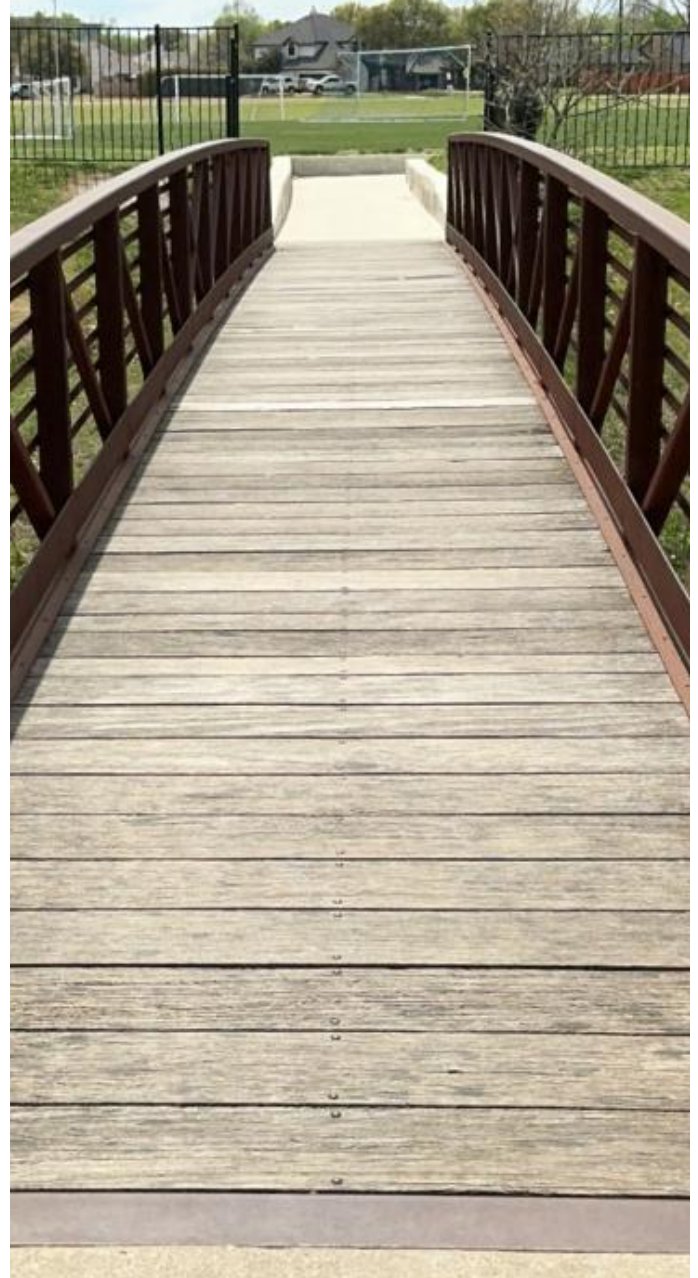
Lakeview Park Trail: Utility Bridge
