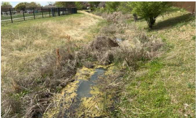
Lakeview Park Trail: Under Utility Bridge
