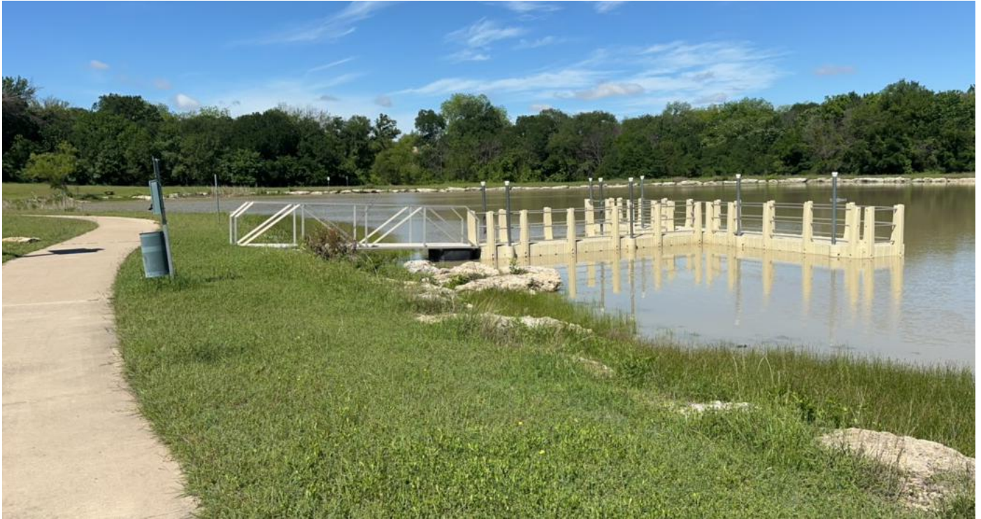
Linear Park: Pier Near Chatswood Drive
