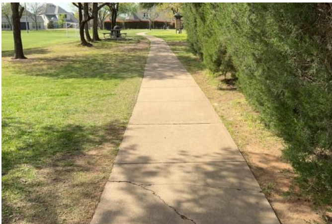
Harmony Park: Perimeter Concrete Sidewalk
