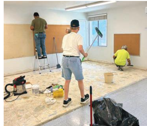
From left, volunteers Gilberto Lira, Martha Shaver, Bill Broadwell, and Peter Lahoo work to renovate a room. (Photo by Gail Haag/Special for Times of San Diego)
