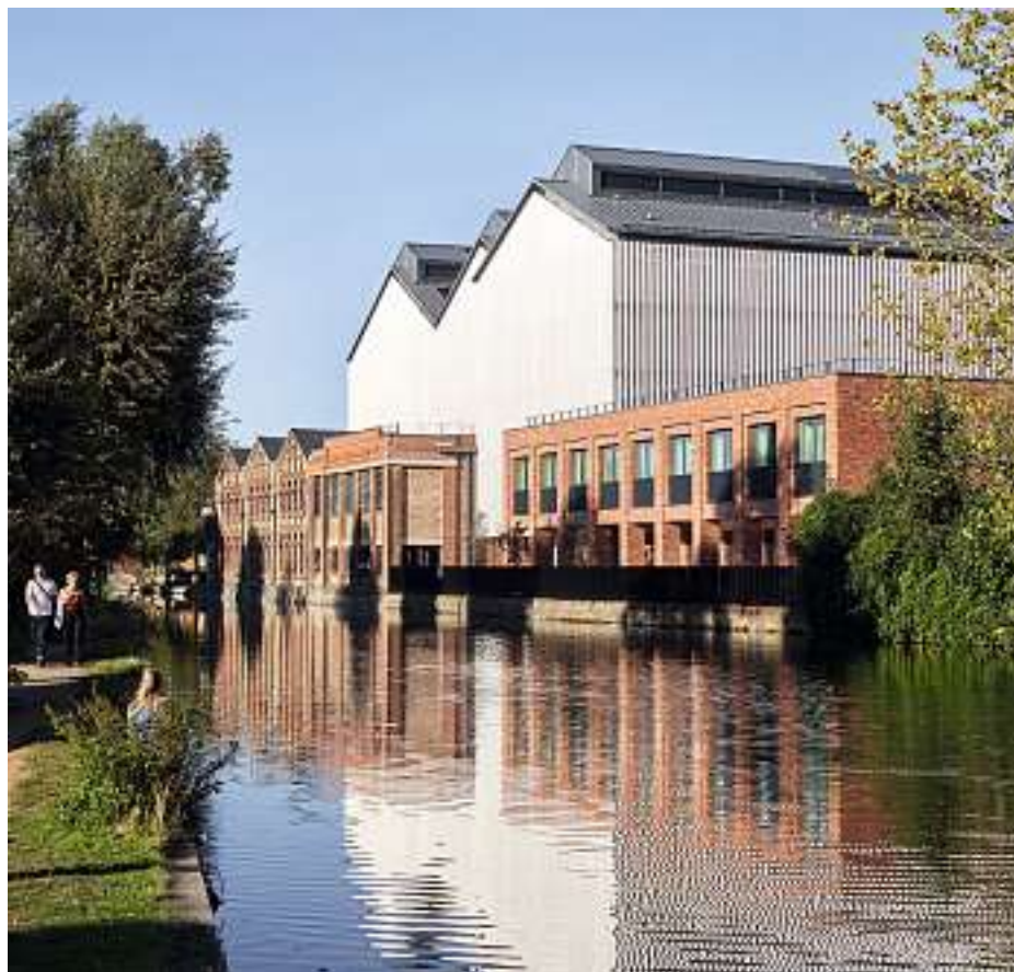
Above: The existing building stripped out.
