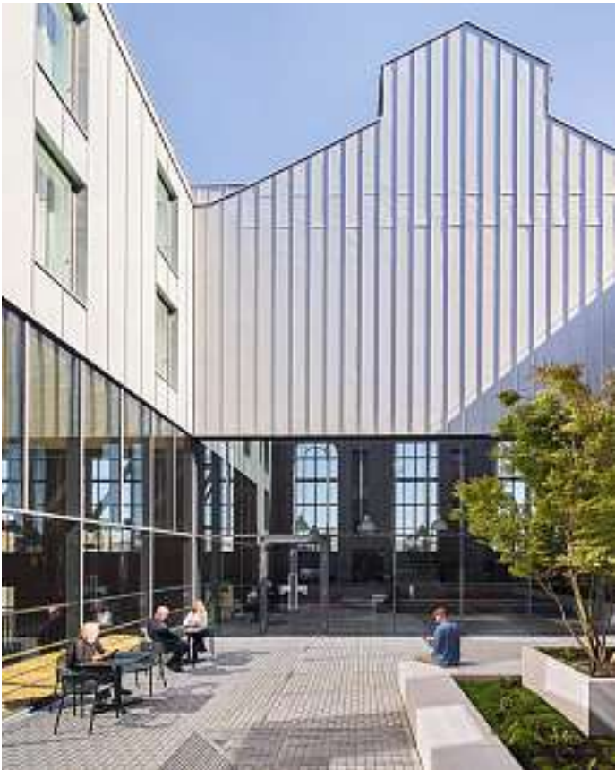
Left: A courtyard set into one of the former turbine sheds draws daylight into the GLC, and adjoins the glass-walled library.
