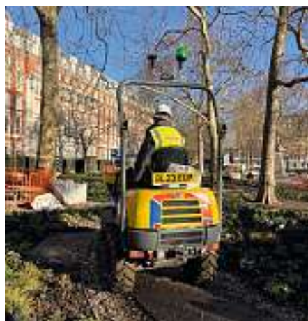
Top left: Screw piles were positioned to avoid tree roots.
