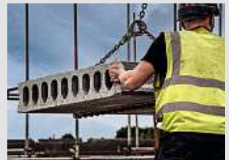
Hollowcore planks can be installed without formwork or propping, helping to simplify construction.
