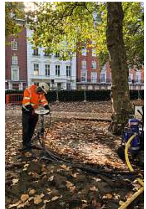
Above: More than 30,000 terraventing holes were made across the site.
