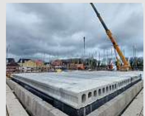
Hollowcore provides a fast, efficient flooring solution across a wide range of building types.
