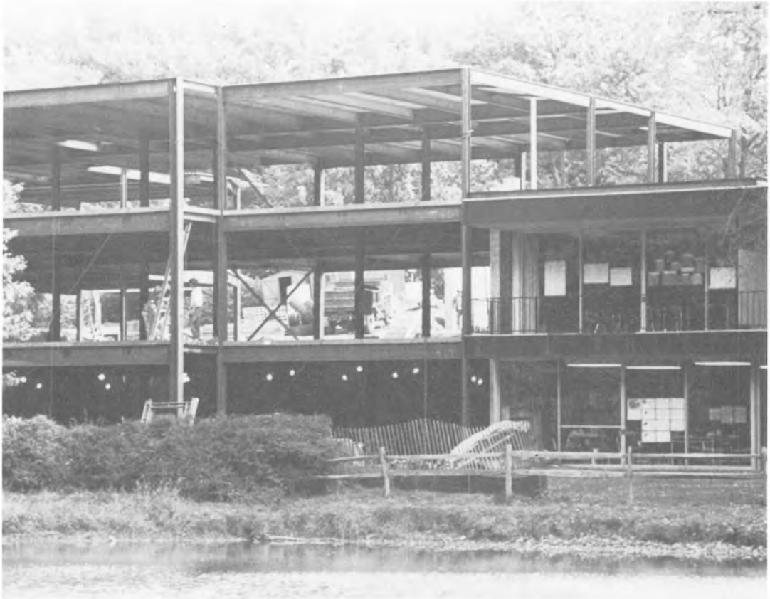
The Academy's new classroom building, shown here under construction, connects the Middle and Lower Schools and provides an attractive and highly functional "bridge" facility, enabling the school to respond with flexibility to future, changing demographics and academic needs.
