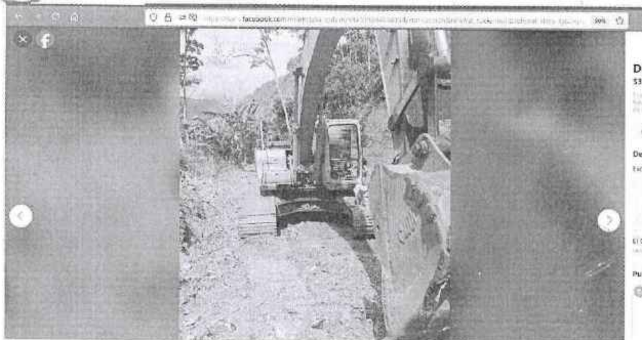
Figura 16 Market place excavadroa doossan
