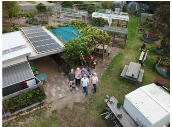
Aireys Inlet Community Garden from above, showing new solar panels
