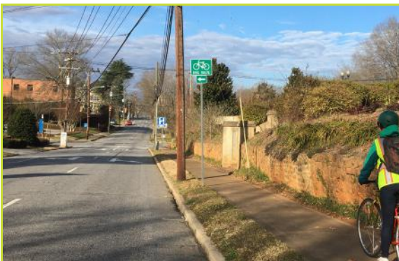
Existing grade and utilities make sidewalk widening or installation challenging in some locations.
