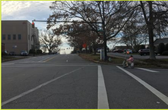
Details such as sidewalk misalignment with the crosswalk are overlooked in certain instances.
