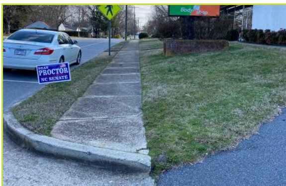
Some sidewalks lack curb ramps and limit accessibility.
