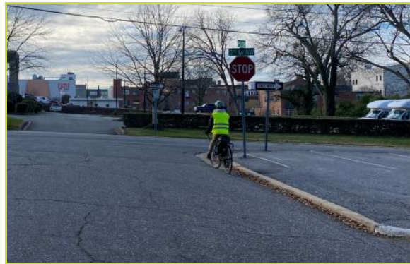
Crossings lack designated pedestrian space. There are unnecessary driveways/curb cuts along many roads.
