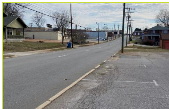
This potential pedestrian space is unclear and fragmented by driveways and utilities.
