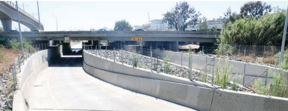
Hazard Center Drive Westerly Expansion. (Photo by Adrian Childress/Times of San Diego)
