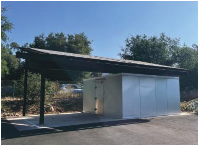
CAUSA Cooler Exterior
