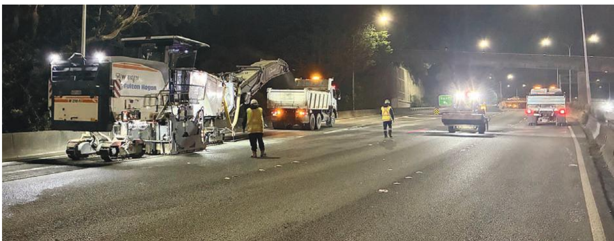
Road resurfacing, which is planned for State Highway 1 on 29 October, taking place. Photo: NZTA/Waka Kotahi.
