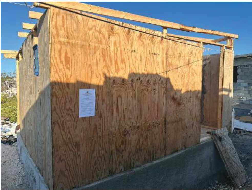
A notice placed on a wooden structure in Five Cays
