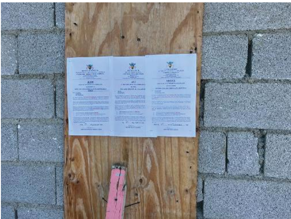
A notice placed on a concrete structure in Five Cays
