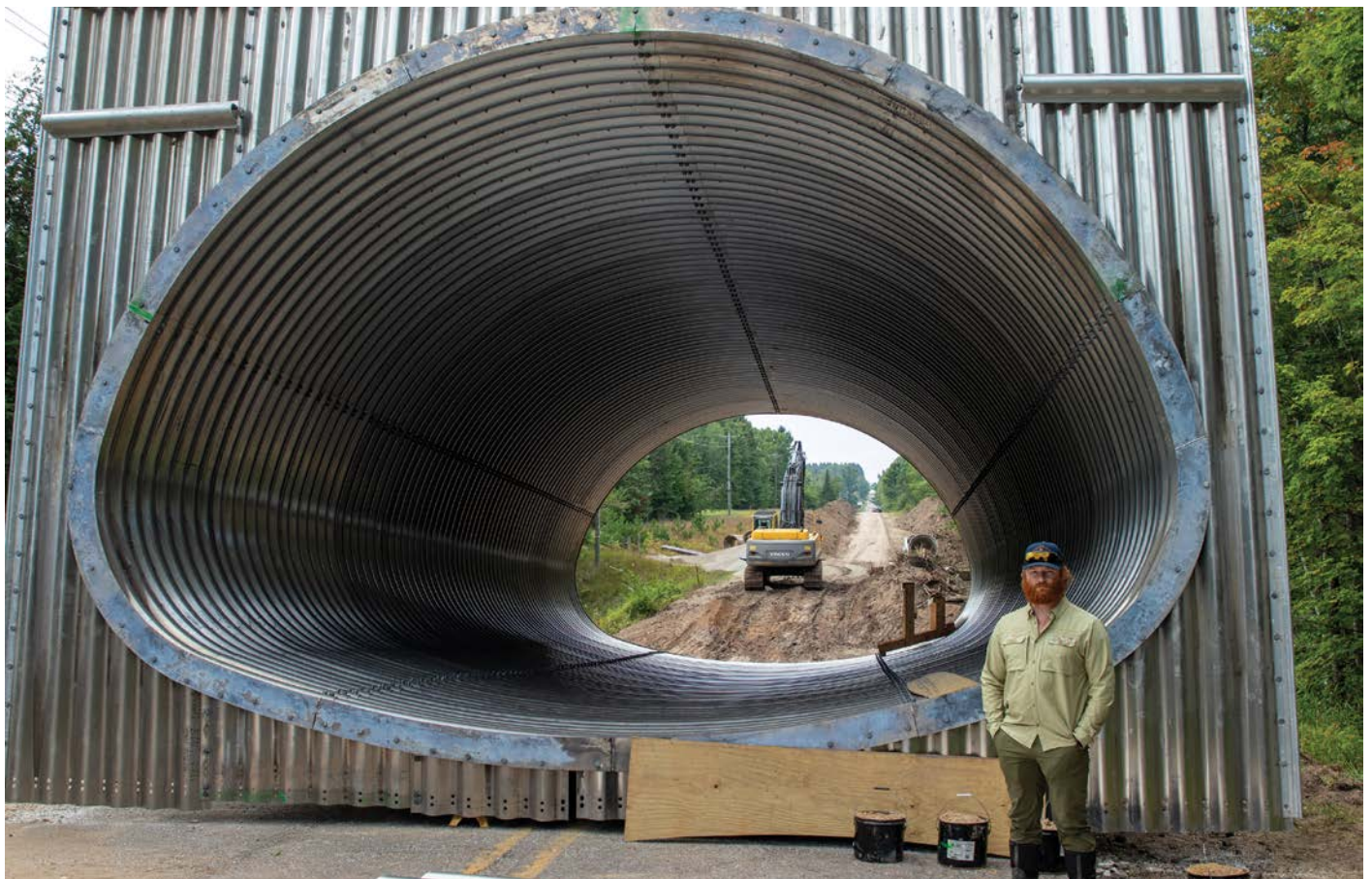
A towering new full-span crossing awaits installation at Maple Creek and Sharon Road.
