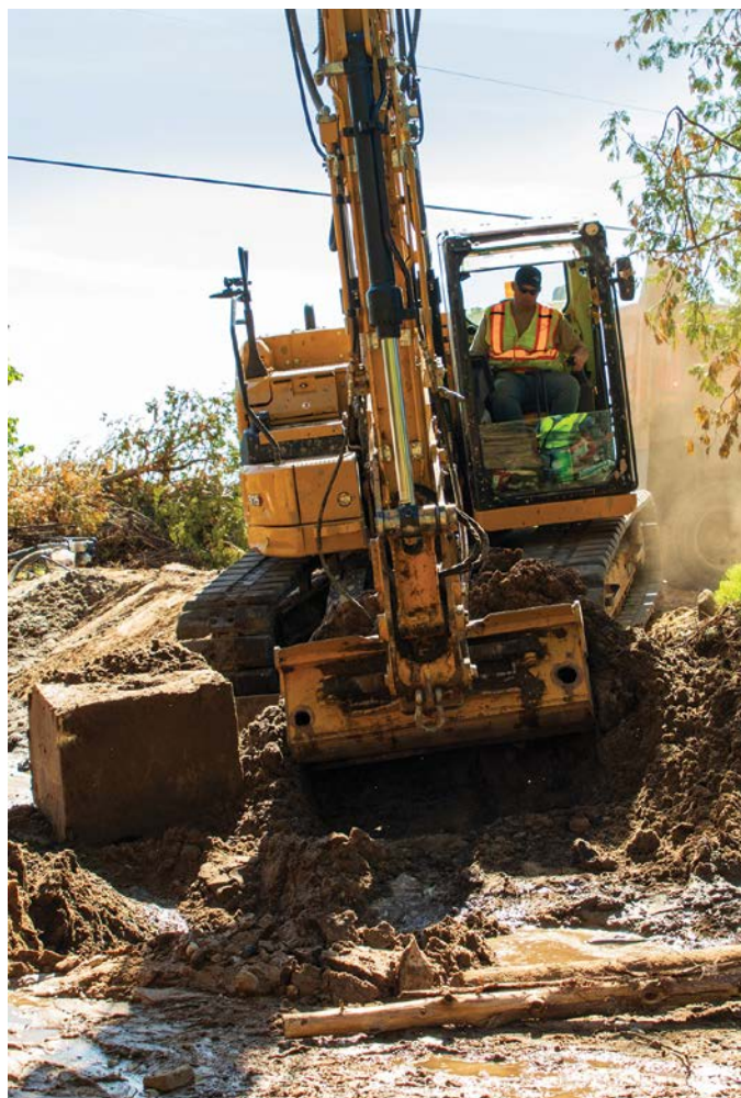
Crews dismantle one of the two dams in June 2026.
