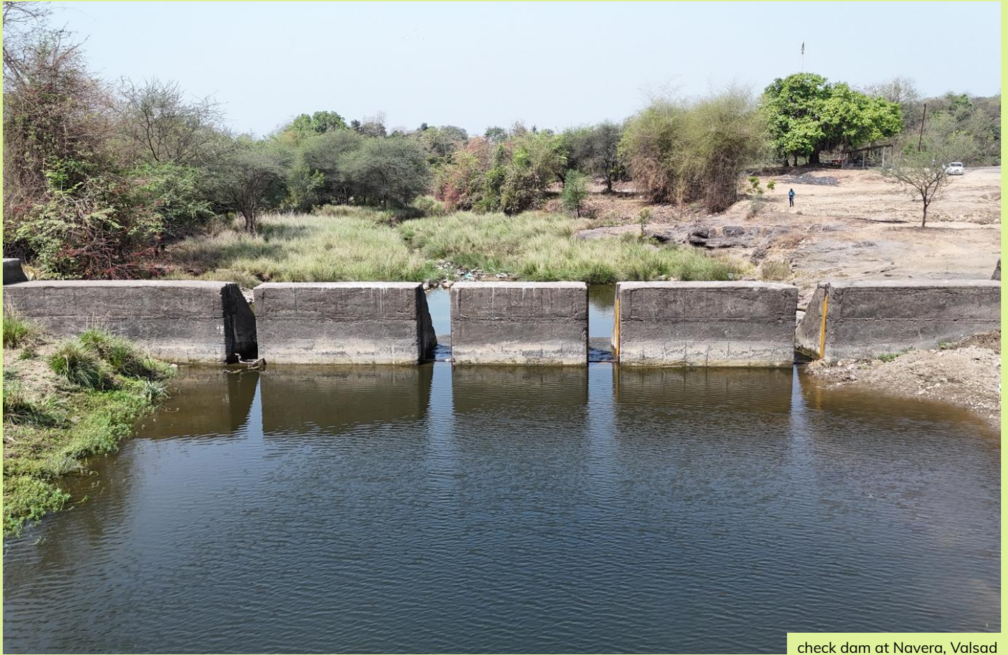
check dam at Navera, Valsad
