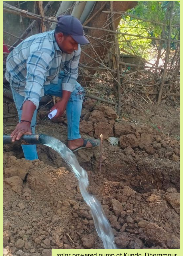
solar powered pump at Kunda, Dharampur
