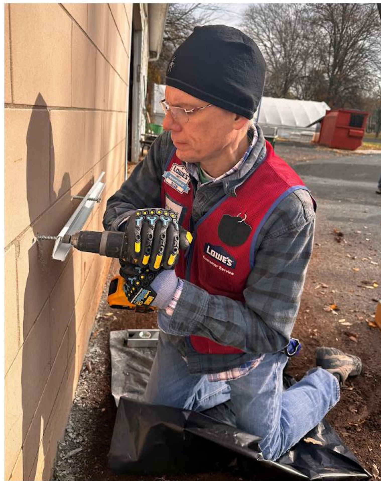
LOWE'S RENOVATES VOCATIONAL CLASSROOMS
