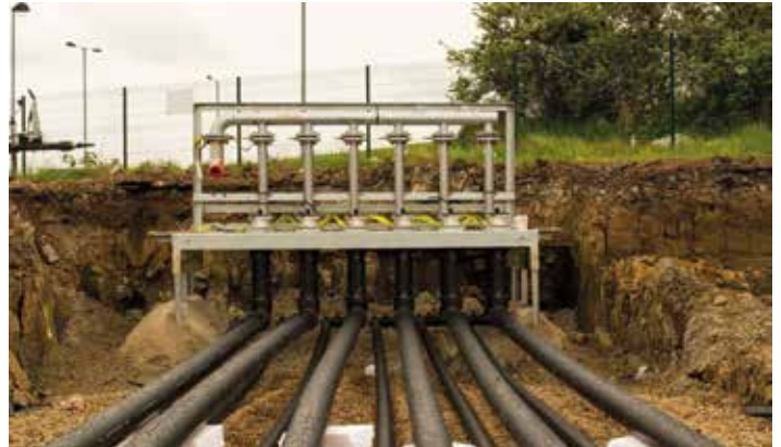
Pipework_PLX_2 - An offset fill arrangement under construction, with PLX pipework runs in position. Fill and vent arrangements are among the first items reviewed when assessing a site for HVO.
