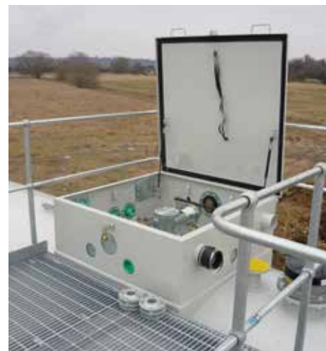
Above_Ground_1 & 2 - A tank top chamber on an above-ground storage installation. Above-ground systems offer greater flexibility as fuel specifications evolve over the coming decade.
