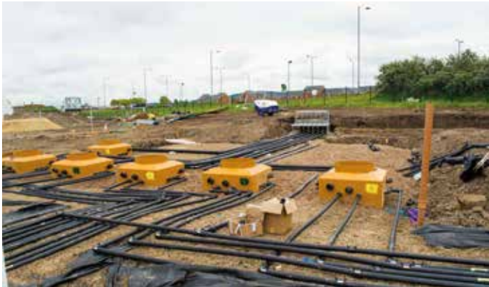
Pipework_PLX_1 - PLX pipework runs and tank chambers in place at a UK forecourt development, prior to backfill. Much of what determines a site's readiness for new fuel grades sits below ground.
