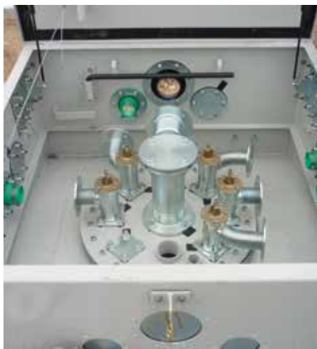
Above_Ground_1 & 2 - A tank top chamber on an above-ground storage installation. Above-ground systems offer greater flexibility as fuel specifications evolve over the coming decade.
