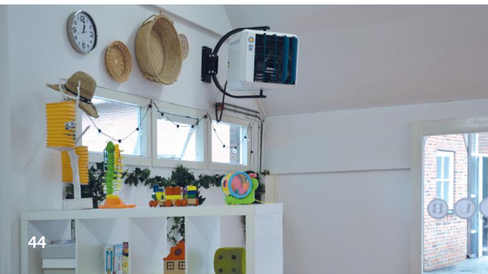
WCU air-circulation unit for improved heat distribution
