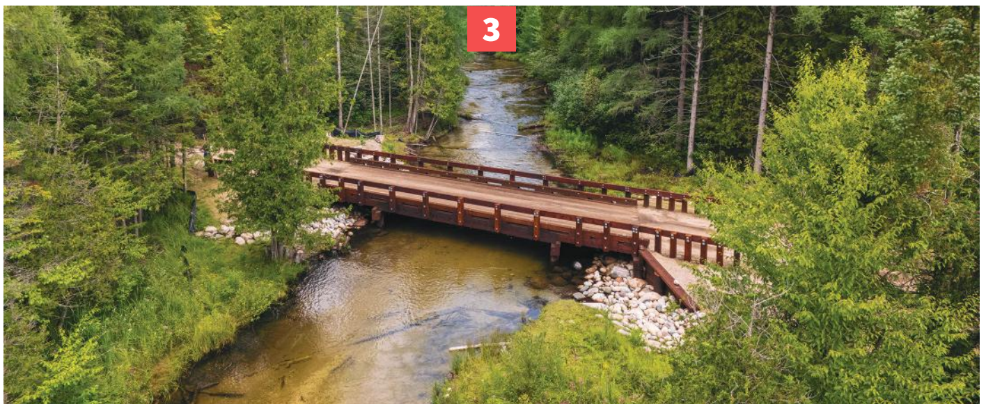
Jordan River and Jordan River Road-West Timber Bridge
