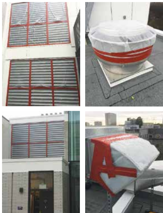
Figure 1: Examples of sealing louvers and mechanical vents for airtightness testing.
