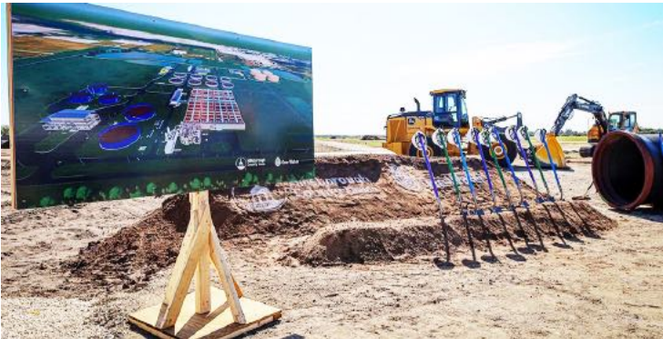
Hillsborough County recently embarked on one of the largest infrastructure projects in the county's history with the $1.2 billion One Water South Wastewater Conveyance and Treatment Project in Lithia.
