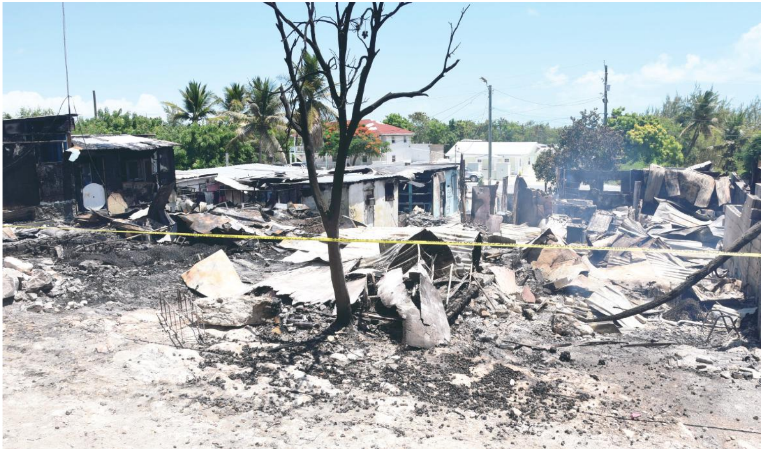
A section of the housing settlement in Five Cays that was razed by fire on Monday, August 24, 2026.
