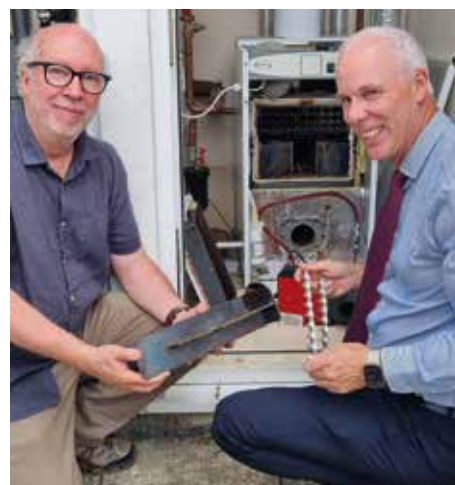
Malcolm Farrow OFTEC and John Weedon Mitchell & Webber admire the cleanliness of the HVO-fuelled boiler.
