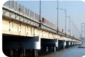
JEMBATAN SURAMADU Suramadu Bridge
