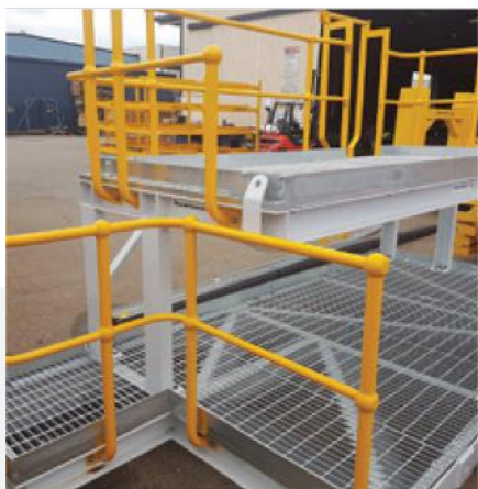
Handrail and Floor Grating
