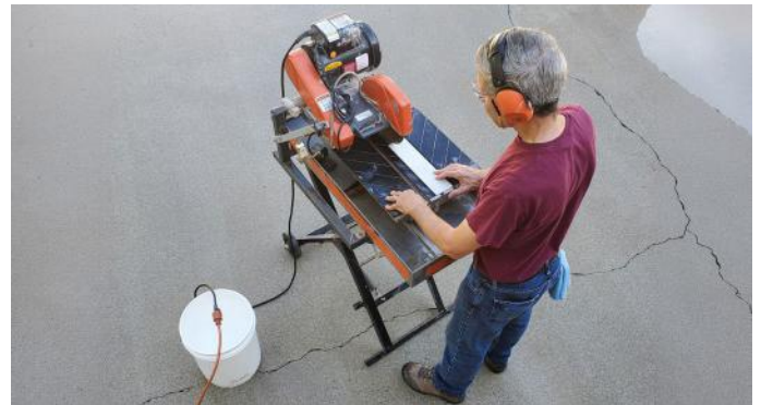
This installer (author Scott Carothers) has the appropriate PPE, safety boots, eye and ear protection, as well as a secure way to keep the extension cord connection safe and dry.
