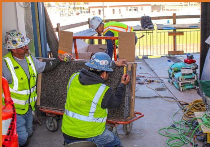
Continental installers measure tile before installation in the Flight Deck VIP Lounge.
