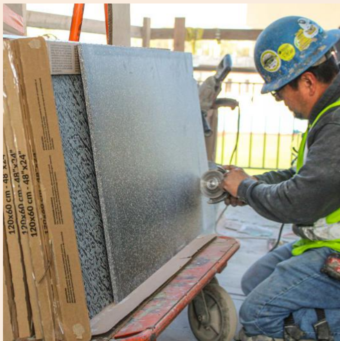
Precise cuts ensured a clean fit around the lounge's architectural details and helped create its unique floor pattern.
