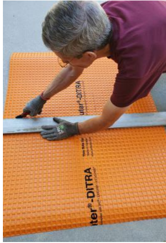
The installer can safely cut materials when protected by ANSI A4 cut gloves, which are mandatory during CTEF training and Certified Tile Installer (CTI) testing.
