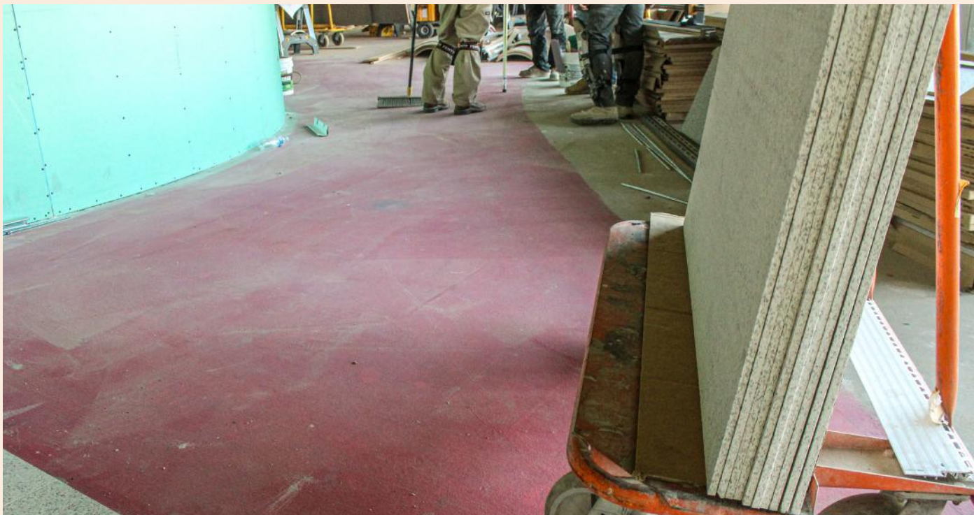
The substrate was prepared with RedGard® Waterproofing and Crack Prevention Membrane before tile installation. In a lounge with a full-service bar, waterproofing reduces the risk of moisture intrusion into the tile assembly.
