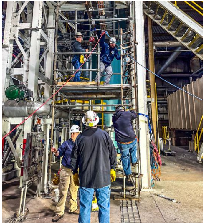
Scaffolding setups demonstrate how to navigate scaffolding safely and how to conduct a rescue if someone falls.
