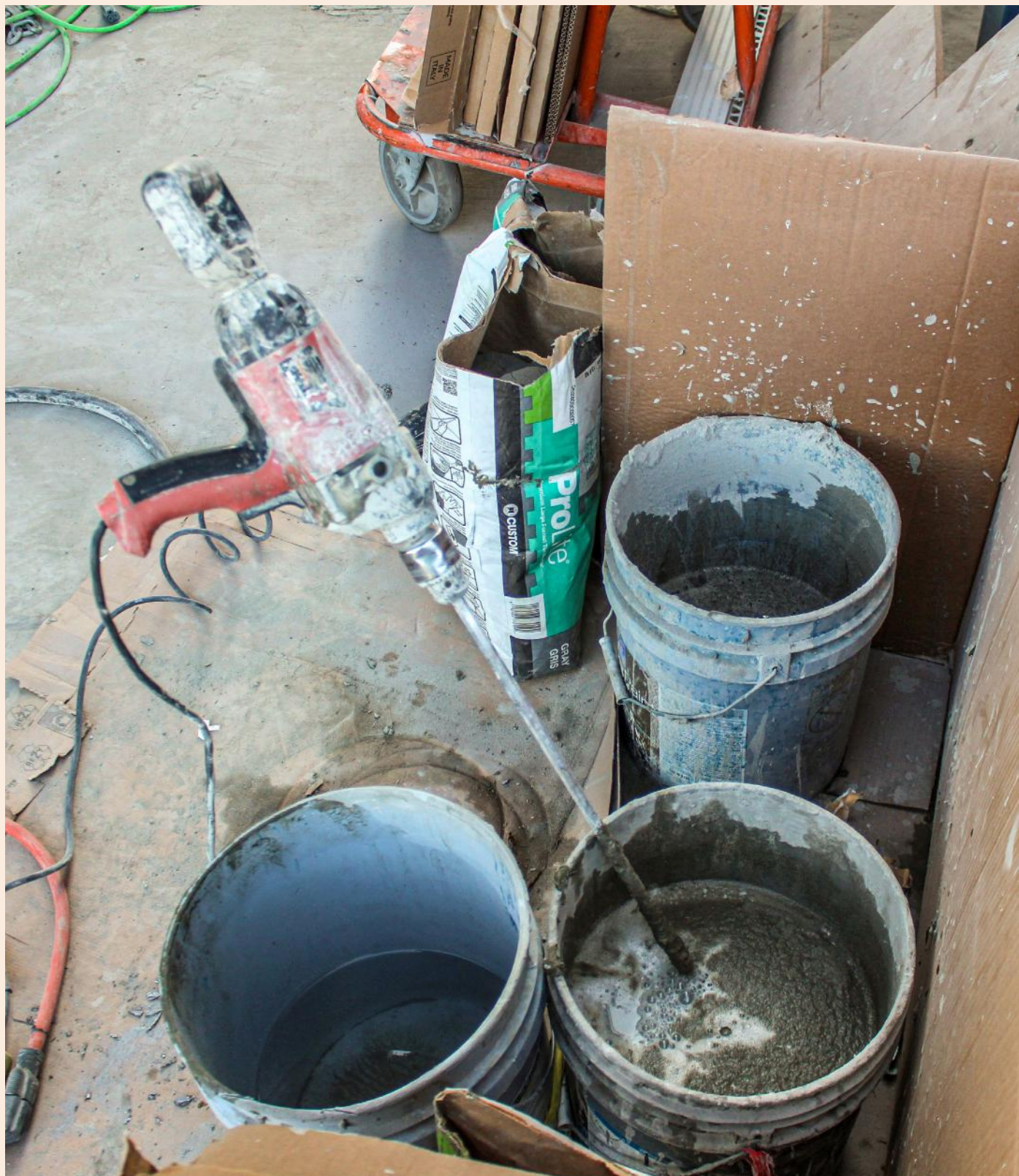
Fresh batches of ProLite® Premium Large Format Tile Mortar were mixed on-site as installation progressed. Its non-sag and non-slump properties made it suitable for most of the tile applications throughout the stadium, including vertical bar tile and large-format floor tile in the lounge.
