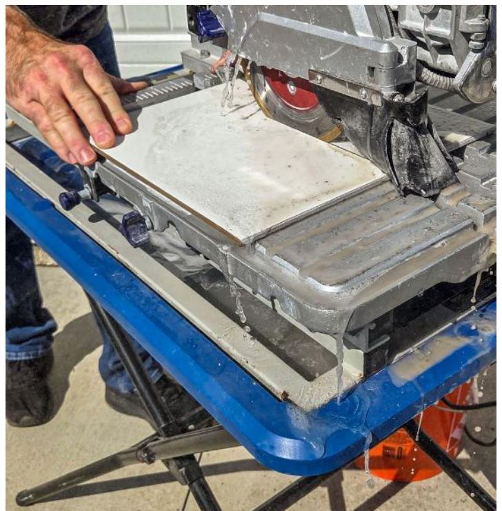
Suppressing the hazard: A continuous-flow wet tile saw effectively suppresses respirable crystalline silica dust at the point of operation.
