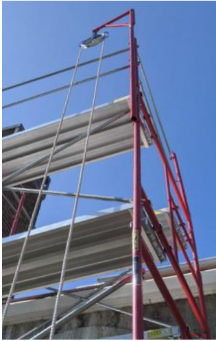
Properly-erected scaffolding provides a stable and safe work environment.
