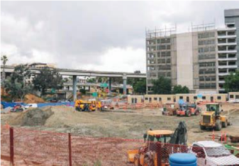
Construction on student housing near San Diego City College. (File photo by Adrian Childress/Times of San Diego)
