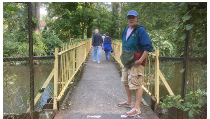
Existing Foot Bridge Across the Chadakoin River, 2023
