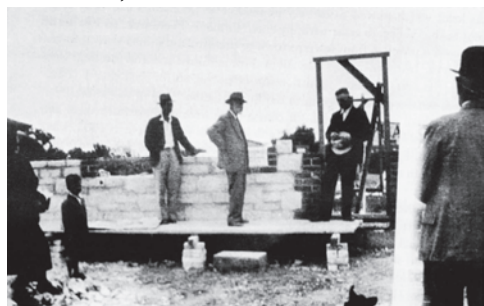
Laying the foundation stone for the Soldiers' Memorial Hall, Second Valley, on 14 October 1922. From left: Charles Roads, Thomas Brown, Captain Hudd, MP (Premier), and James Cussion. The woman and child are unknown.
