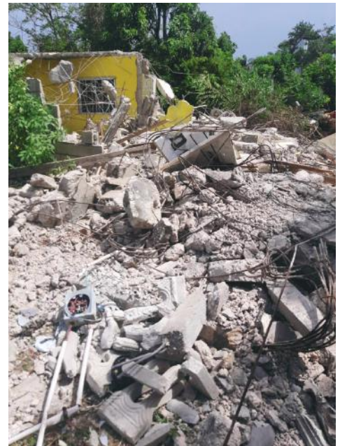
A section of the on which houses were bulldozed
