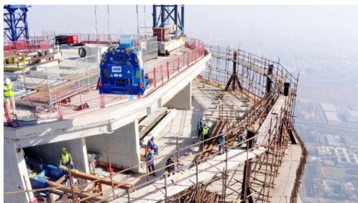
An Otis SkyMotion™ machine, which powers the Otis SkyRise elevator, is hoisted onto the Tianjin 117 Tower; image courtesy of Otis.
