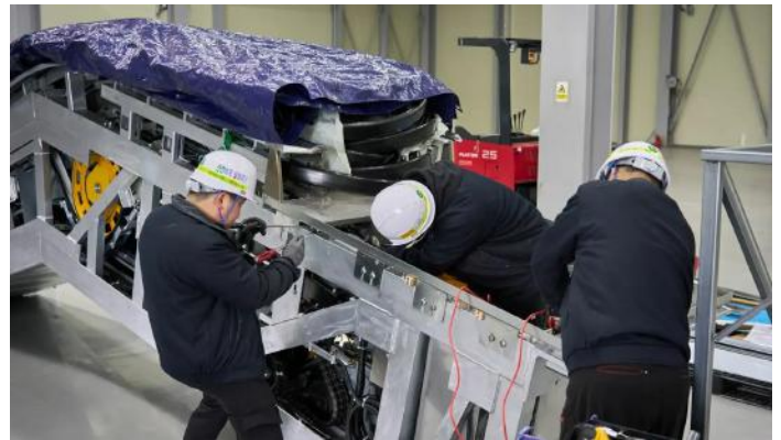
Employees assemble an escalator at K-Escalator's factory in Geochang County, South Gyeongsang; image courtesy of K-Escalator.
