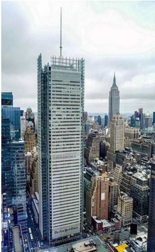
The 52-story New York Times Building in NYC
