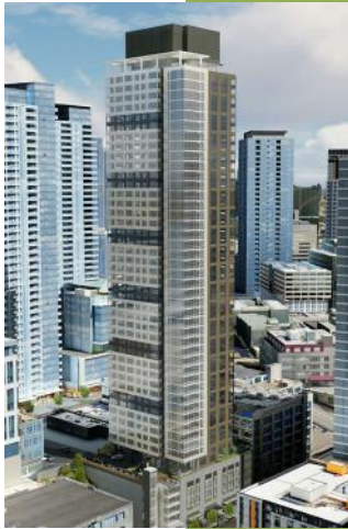
1001 John - Seattle, WA [400 foot, 430 unit residential tower]
