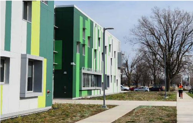
FIGURE 1-16 South Parkway - Before
