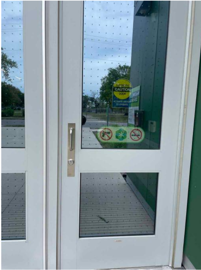
FIGURE 4-03 No Smoking signs at South door
