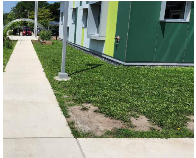
FIGURE 1-15 Evidence of severe foot traffic
