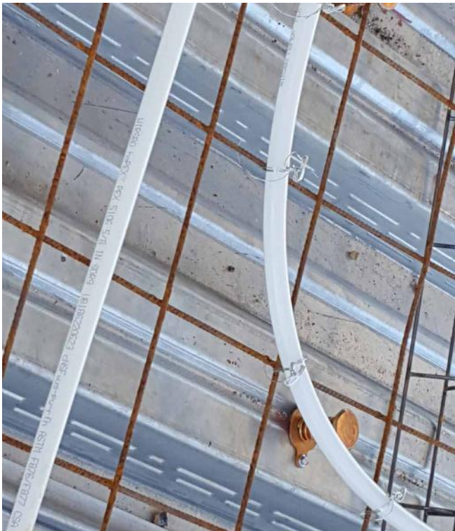
FIGURE 3-18 Detail of Radiant Tubing
