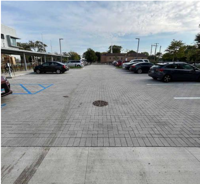
FIGURE 1-52 Pervious Surface Parking
