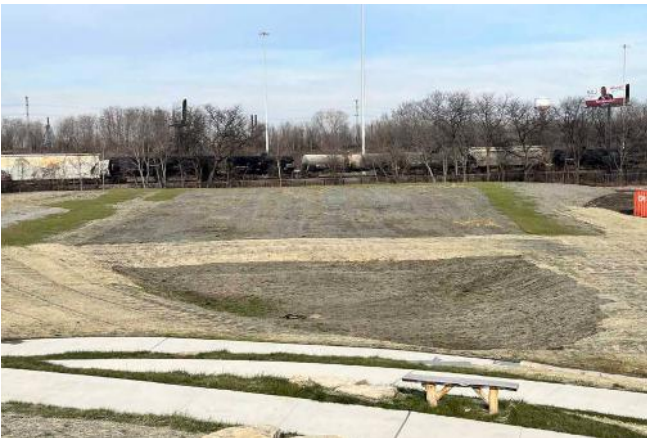
FIGURE 1-17 View Looking North - Before
