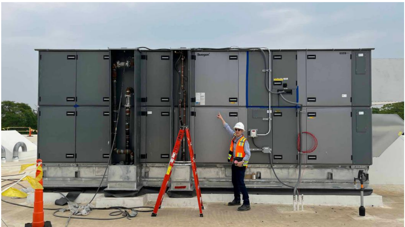
FIGURE 3-14 Our Direct Outdoor Air System
