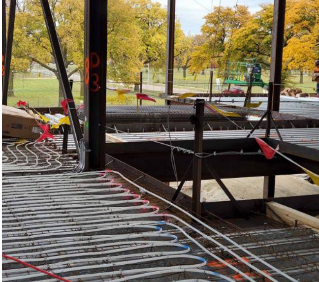
FIGURE 3-13 Radiant Tubing before Concrete Floor
