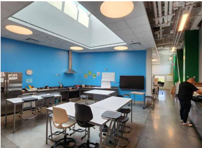
FIGURE 4-16 Skylights bring in natural light to interior areas
