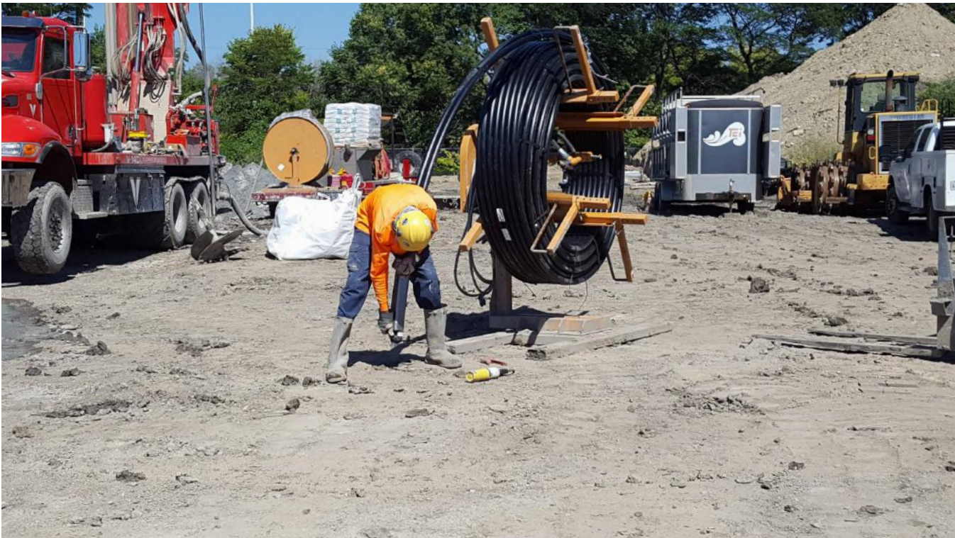
FIGURE 3-16 Geothermal well field install
