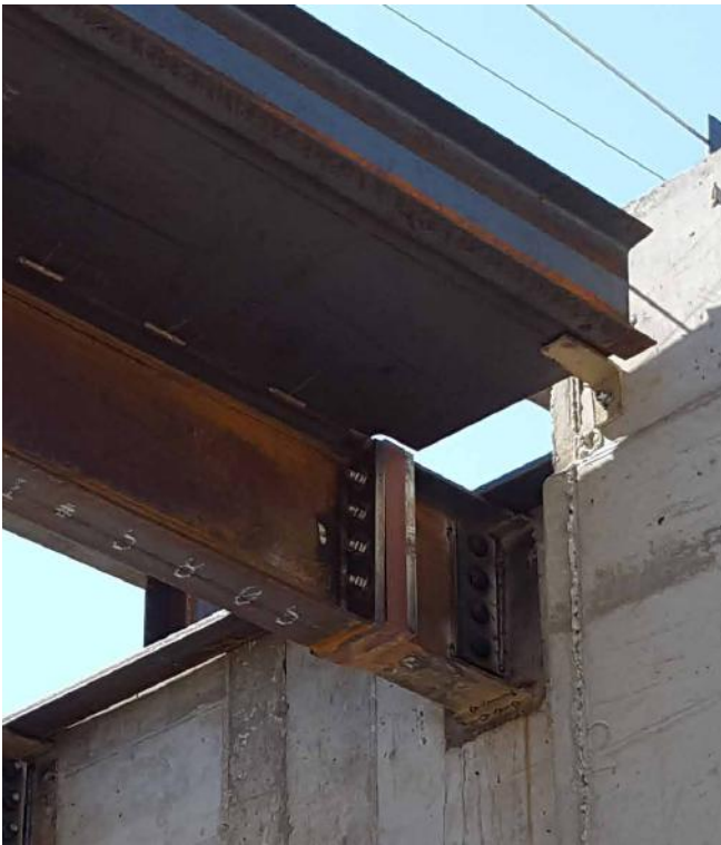
FIGURE 3-17 Thermally broken steel detail
