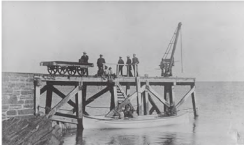
Jetty wagons could be hand pushed at Second Valley, with no need for a horse or locomotive Photo courtesy: Dept. of Marine and Harbours
