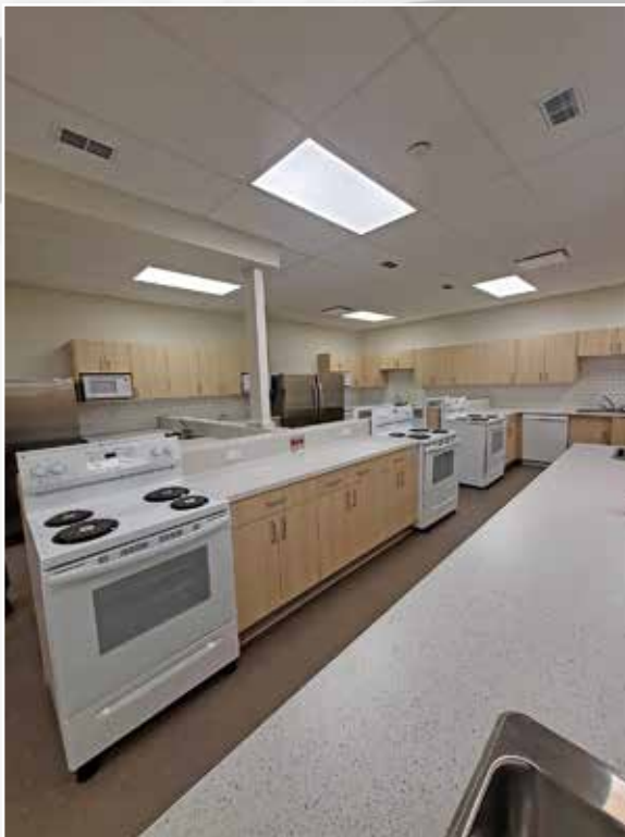
Immanuel Christian Secondary School Home Ec Room Renovation. Ward Bros. Construction Ltd.
