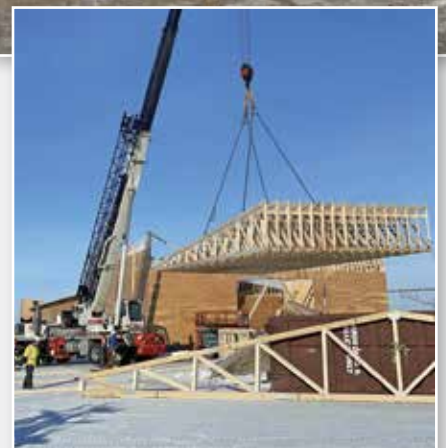
New Way Irrigation. Southwest Design & Construction Ltd.
