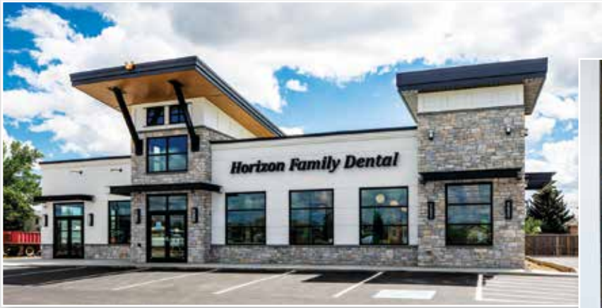
Horizon Family Dental. Southwest Design & Construction Ltd.
