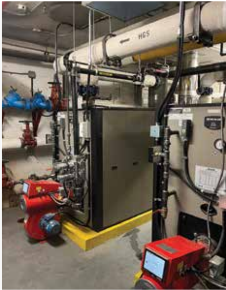
Fritz Sick Pool Boiler Replacement. DMT Mechanical Ltd.
