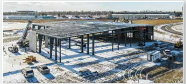
College Ford. Southwest Design & Construction Ltd.
