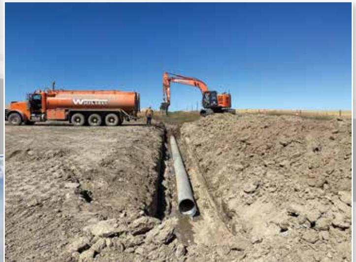
Hilda Project. Whissell Contracting Ltd.
