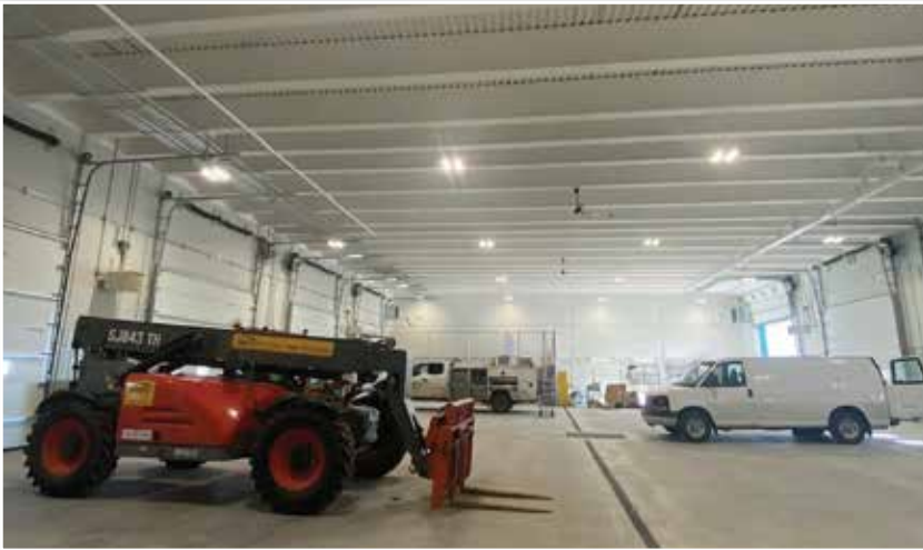
Fortis Garage. Neu-Lite Electric Inc.
