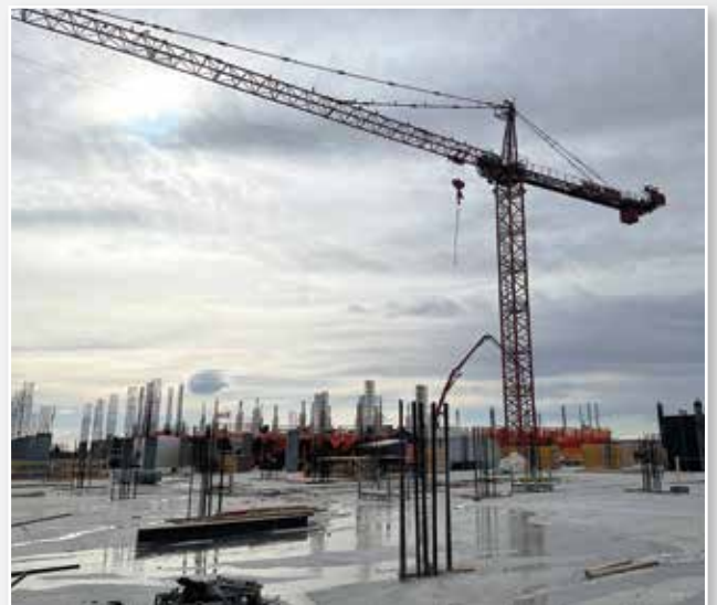
102 Scenic Condos. Phase One Construction.
