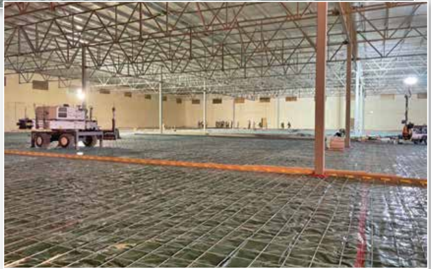
Superform ICF Facility. Link Builders.
