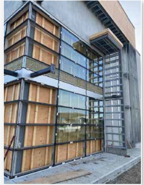
JWB Building. Ward Bros. Construction Ltd.
