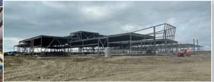
New Coaldale High School and Rec Centre. Ward Bros. Construction Ltd.
