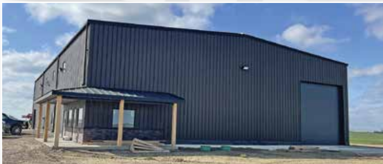
Windland Shop. Southwest Design & Construction Ltd.
