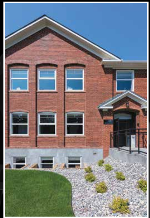
Abbey Road, Phase 1. Photo courtesy of Silver Ridge Construction
