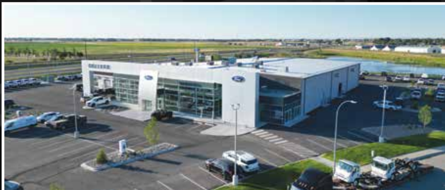
College Ford Lincoln. Photo courtesy of Southwest Design & Construction.
