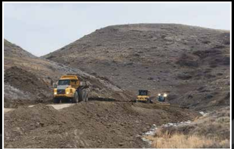
Coulee spillway haul road building.
