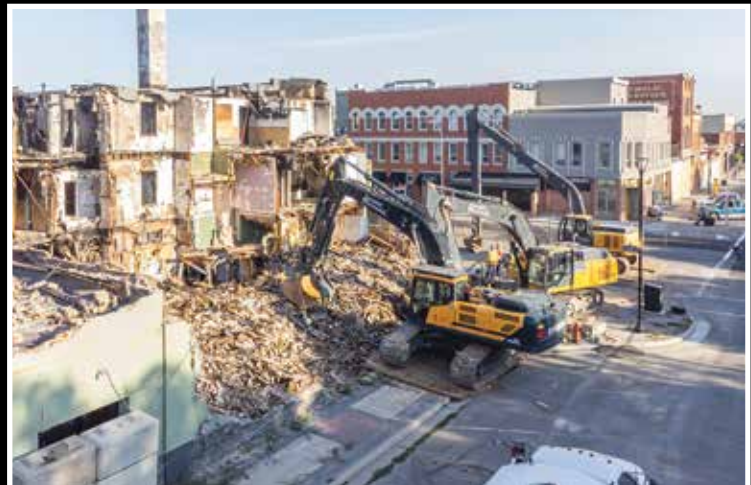
Lethbridge Hotel demolition in Lethbridge. Photo courtesy of Dennis Dirtworx Ltd.
