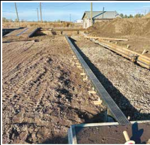
Poly Trench Drain in Taber, AB.
