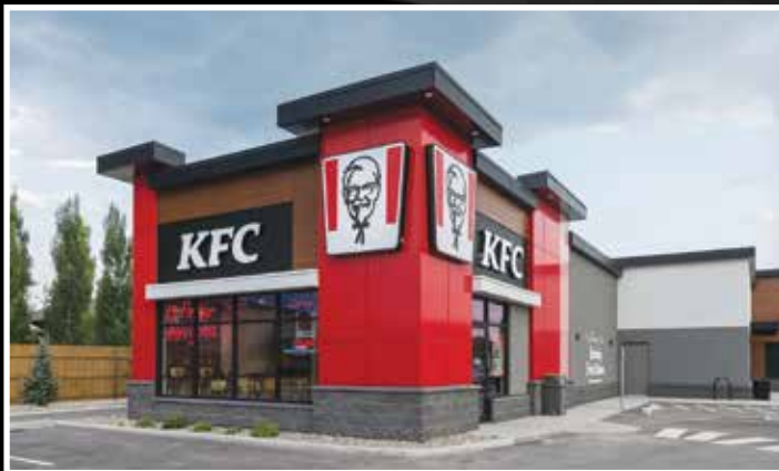
KFC Coaldale. Photo courtesy of Silver Ridge Construction.
