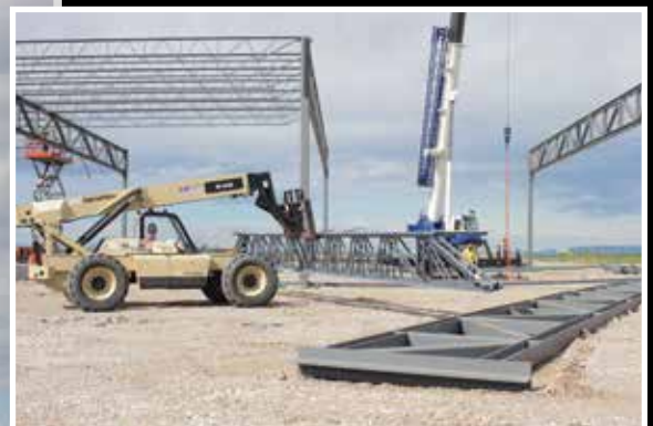
Structural Truss Forma Steel.
