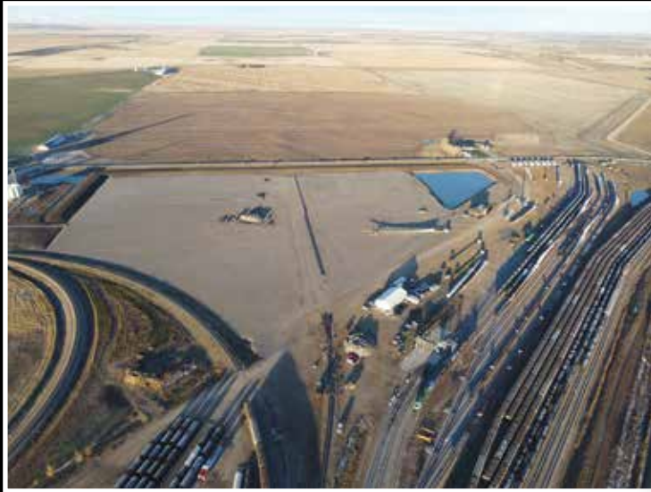
Gravel placement for wind turbine laydown. Photo courtesy of McNally Contractors (2011) Ltd.
