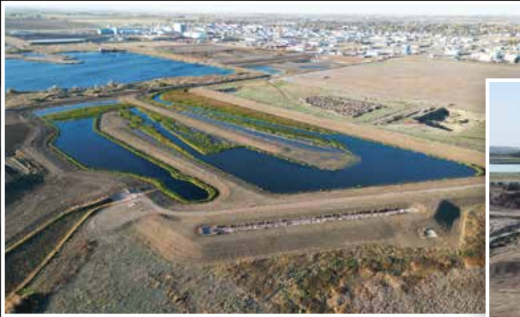
Taber wetland complete. Photo courtesy of deGraaf Excavating Ltd.
