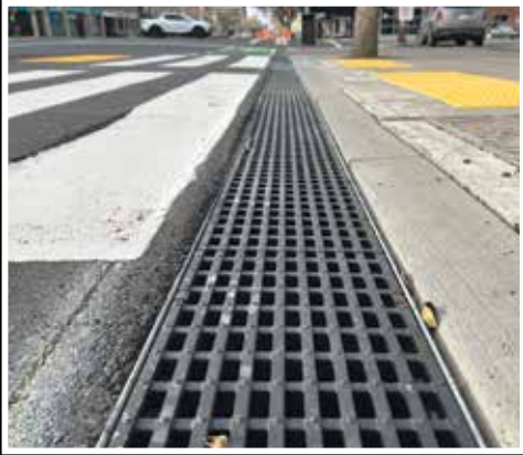
Trench drain and two tactile plates at transit stop in Lethbridge.
