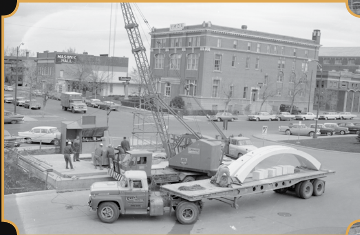
1963-A truck delivers the sections for the arch of the Memorial to the Pioneers of Irrigation in downtown Lethbridge.
