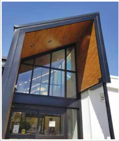
Red Deer Recovery Community. Photo courtesy of FWBA Architects.
