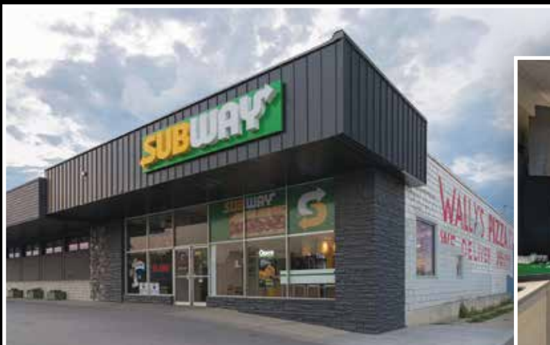
Subway in Coaldale. Photos courtesy of Silver Ridge Construction.
