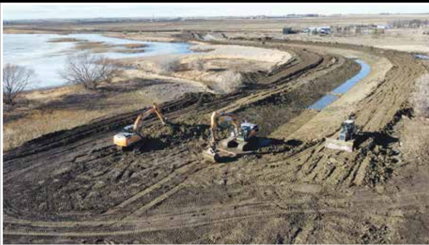
Lethbridge Northern Irrigation District, Picture Butte Reservoir Diversion Channel.
