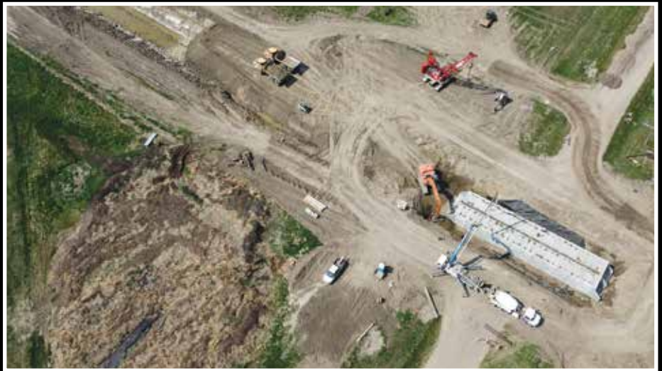
Box culvert backfill.
