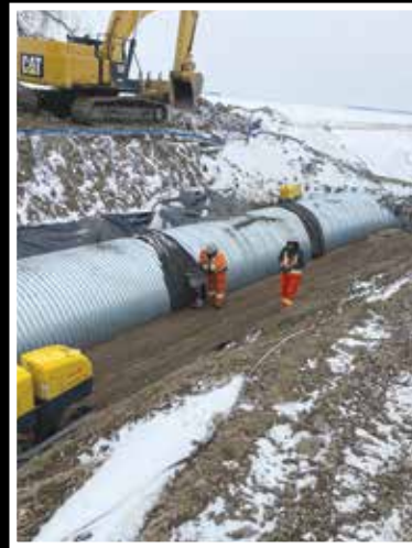
Large diameter gravel road bridge culvert installation for drainage canal. Photo courtesy of McNally Contractors (2011) Ltd.
