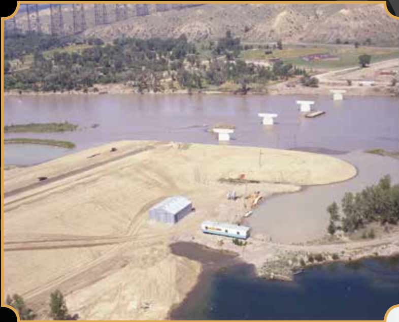
July 1974 - View of the construction of the Whoop-Up Drive Bridge.
