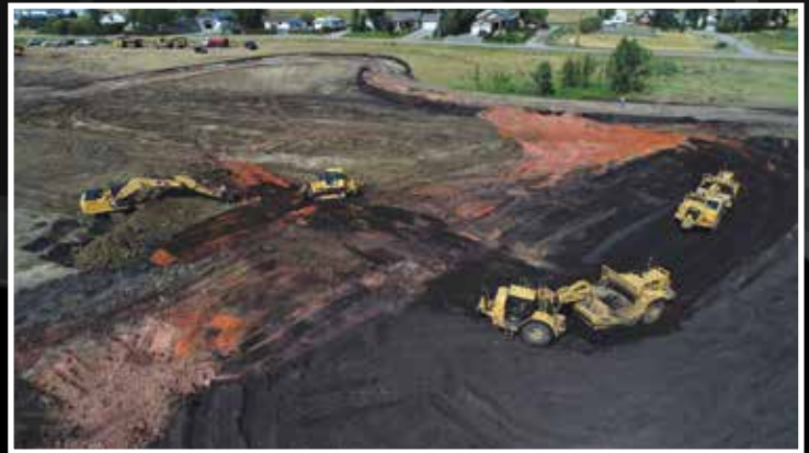
Excavation of wetland on the Town of Coalhurst Main Constructed Wetlands. Photo courtesy of McNally Contractors (2011) Ltd.
