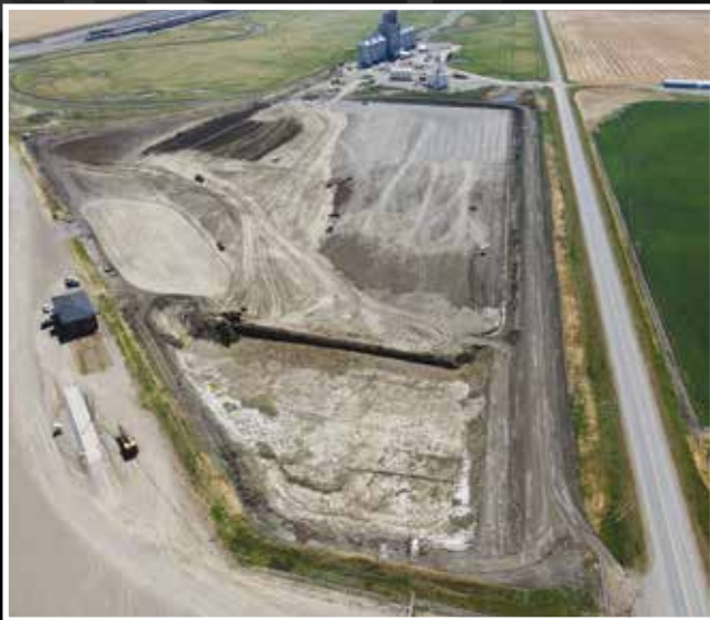
Gravel placement for wind turbine laydown. Photo courtesy of McNally Contractors (2011) Ltd.
