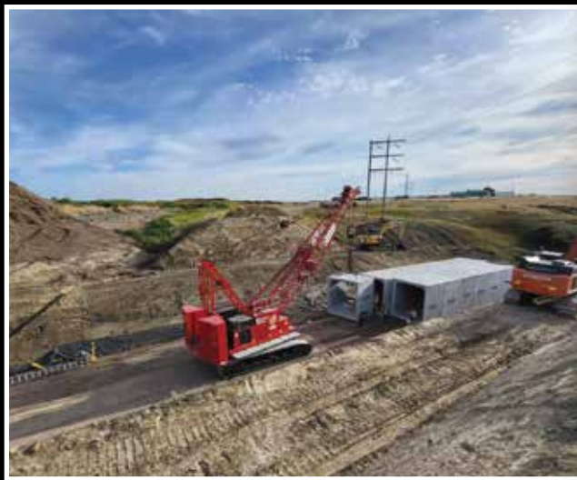
Box culvert placement.
