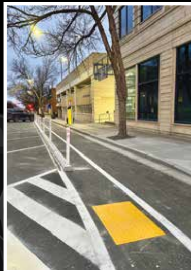
Bicycle lanes in Lethbridge. Delineators and two tactile plates. Photo courtesy of CT Distributors Inc.
