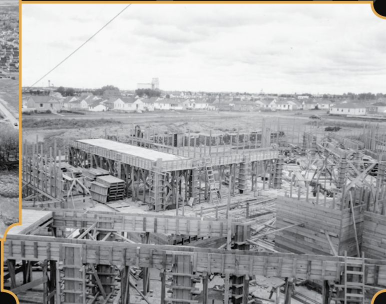
December 1953 - Showing the construction of the Municipal Hospital 9th Avenue and 18th Street South.
