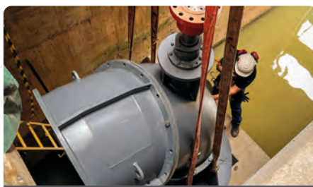
PROJETO DIQUE SANTA CLARA – 3SB BLUMENAU - SC
