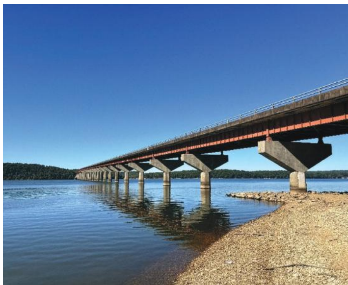
Fig. 1: Puente John Coffee Memorial
