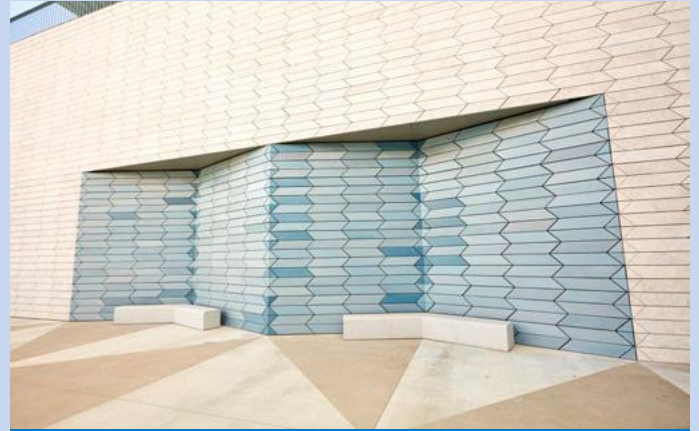
Intricate architectural details throughout the Ismaili Center reflect the close collaboration among designers, installers, and MAPEI technical experts.
