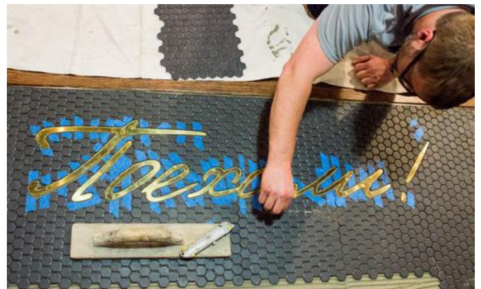
Trexel designed and installed this piece for the owner of Kachka restaurant five years ago. He sourced the brass and commissioned a waterjet-cut brass inlay for the lettering, then finished the unique and challenging project with epoxy grout.
