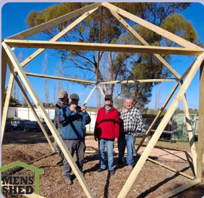
Star Plate Geo Dome built by Red Cliffs Men's Shed members for The Red Cliffs Grow & Share Garden.
