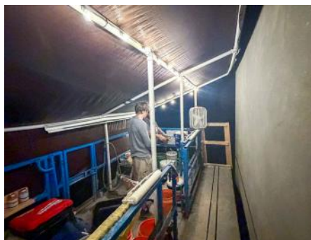
Working at night.
