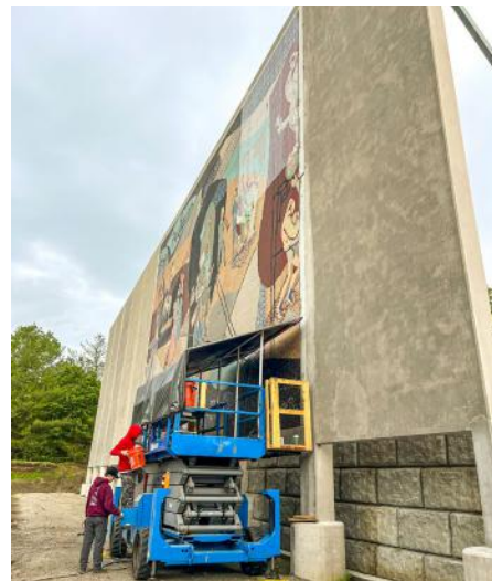
Prepping a section for grout. Removing tape and draping squeeze through.
