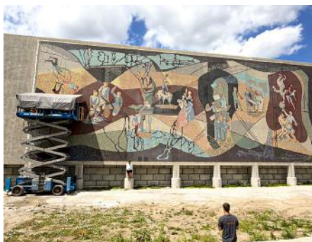
Progress photo with lift.
