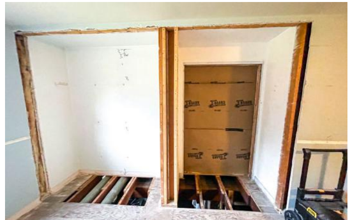
Former bedroom after demo. Two closets were removed to make room for a shower and a water closet. The subfloor is 1/2" plywood on 16" OC 2"x 8" joists. The subfloor was not flat under the former closet floors due to floor joists overlapping at the carrier beam. The structure had sagged and the joist ends were not properly fastened at the time of original installation, so over time they pushed up on the subfloor and created high spots.
