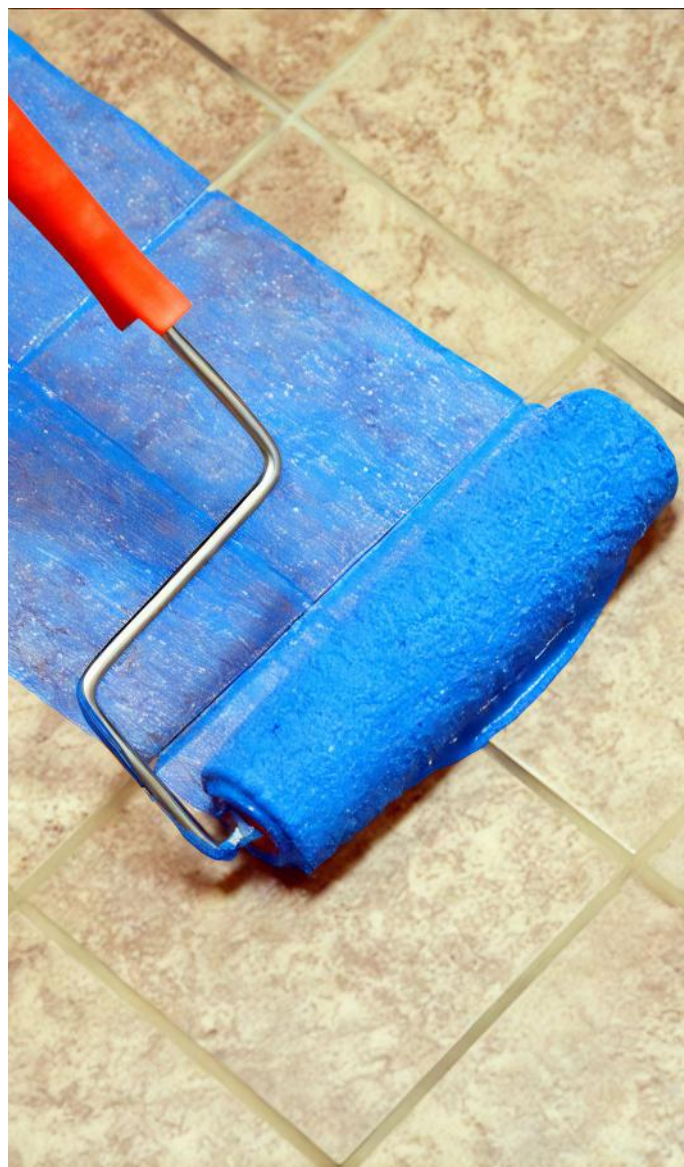
A bonding primer or mechanical abrasion may be recommended to improve the bonding surface of existing tile to prepare for a tile-over-tile install.
