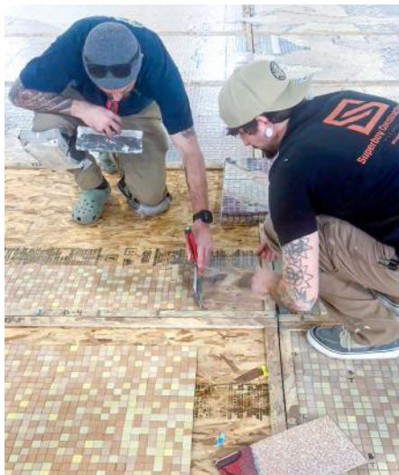
Returning desheathed tile to its plywood staging sheet.
