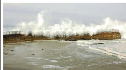
A huge wave rolls over the seawall protecting the Children's Pool.
