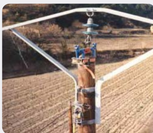
Readjusting the height of a post fitting
