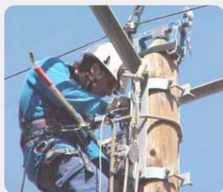
Positioning on top of wooden post
