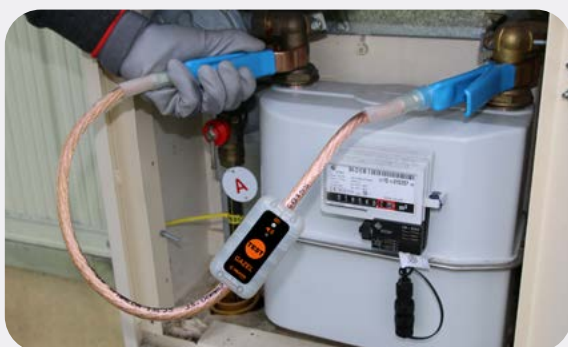
3 THE BYPASS MAINTAINS THE CONTINUITY WHEN THE OLD GAS METER IS REMOVING TO AVOID ANY SPARK
